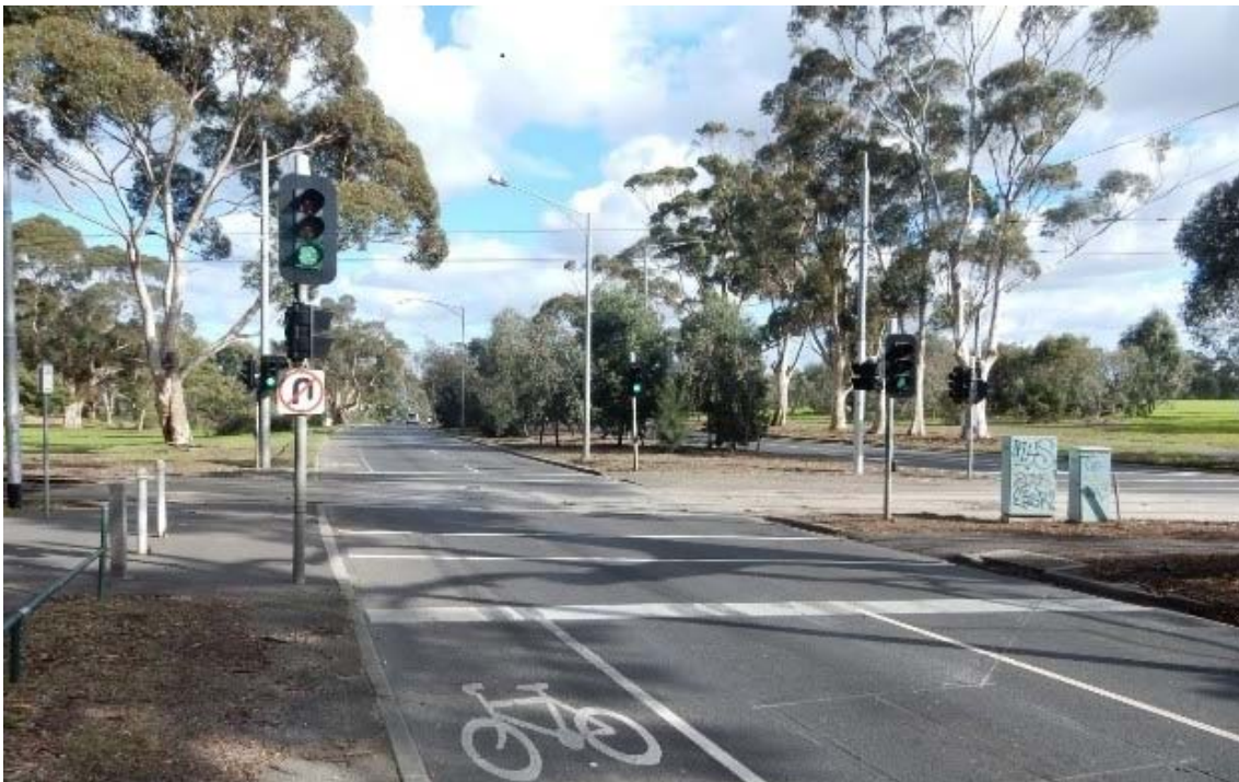
Figure 5: Road traffic lights on the east-to-west carriageway (the carriageway used by the truck).
