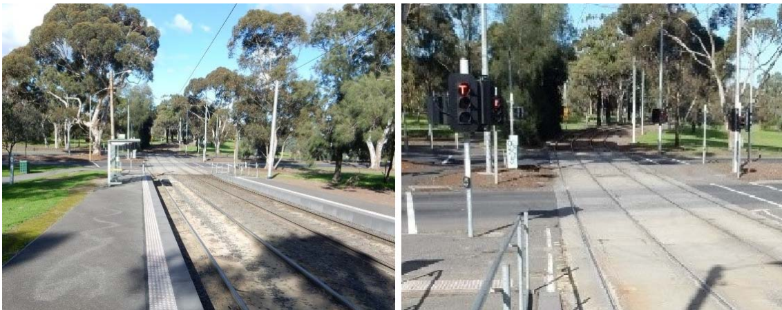
Figure 6: Tram approach to Elliot Avenue from the North - the tram stop (left) and 'T' light (right)
