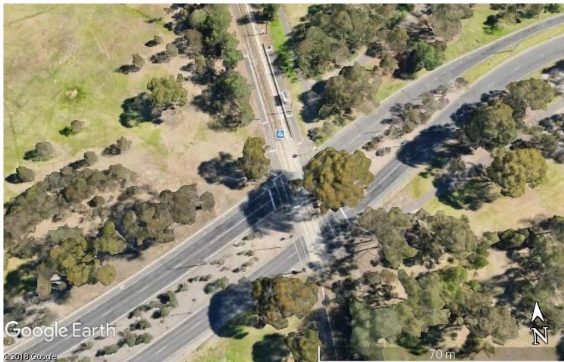
Figure 3: Aerial view of the tramway crossing of Elliott Avenue
